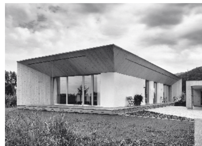
Architect Georg Bechter used straw as an insulating material for the straw house in Dornbirn and also for the supporting structure.
